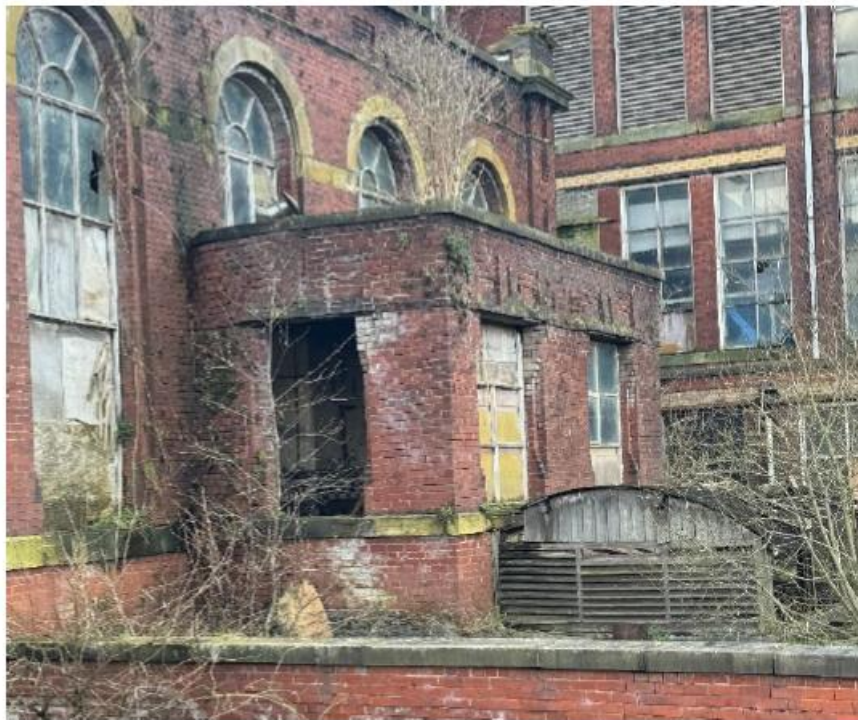
Figure 18 – Photograph of Engine Room Extension
