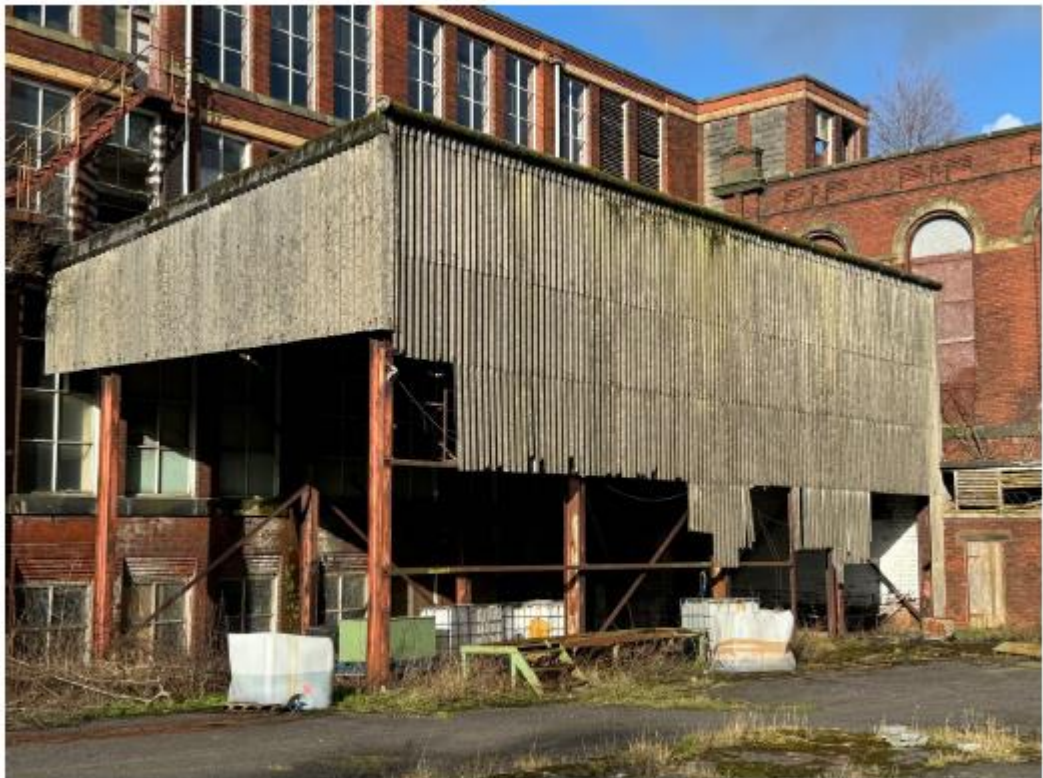
Figure 23 – Photograph of Steel Structure
