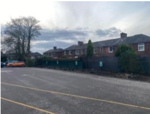
Rear elevations of some of the properties on Emerald Ave (above)
